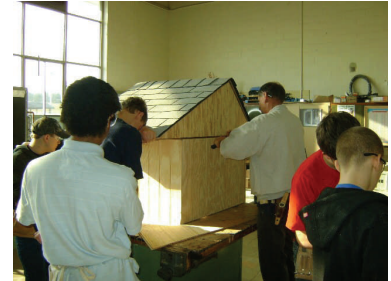
Ms. Stano's Carpentry shop students are building a dog house.
